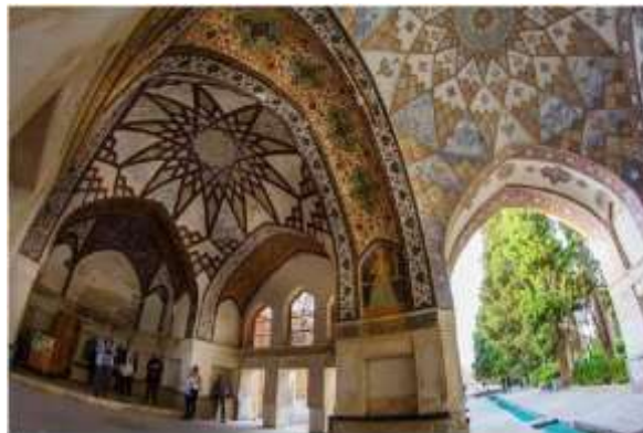
Fig. 5. Ceiling of the kushk: A 12-sided star with angular extensions on the Kushk.
