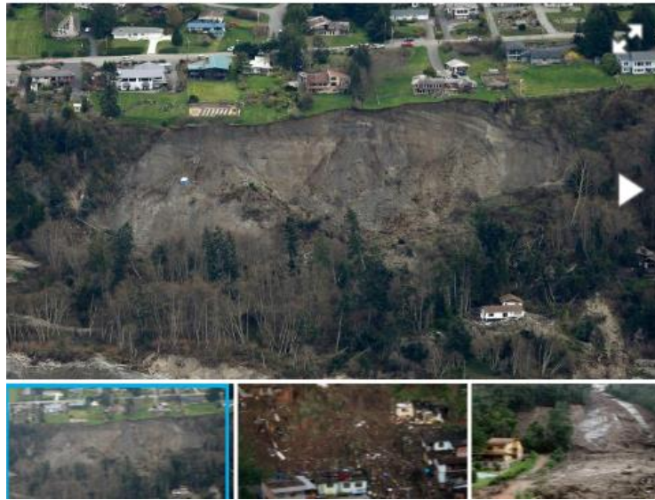
Rice. 1. Collapse caused by natural causes.
