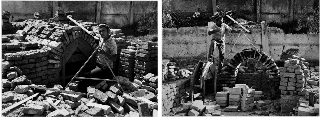
Photo 1. Measurement of the arched firebox opening of the khumdan in Shakhrisabz. The photograph documents the measurement of the arched opening during the construction and testing of the kiln. Archival photograph, 1980s.
