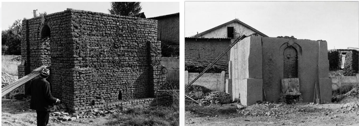
Photo 2. Construction and reconstruction of a brick khumdan kiln in Shakhrisabz. The photograph documents the process of erecting the walls and structural components of the kiln. Archival photograph, 1980s.
